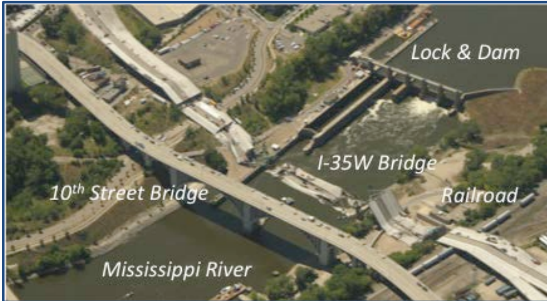
Photo 2: The collapsed bridge and surrounding area on 2 August 2007. Photo courtesy of the Minnesota Department of Transportation.
