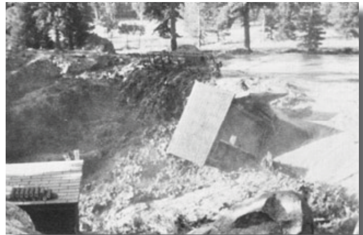
Lawn Lake Dam failure, Colorado. 1982
