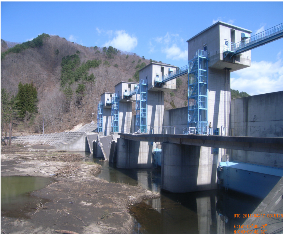
Seawall gate protected Fudai in Iwate Prefecture despite being overtopped. Photo courtesy of Gary Chock.
