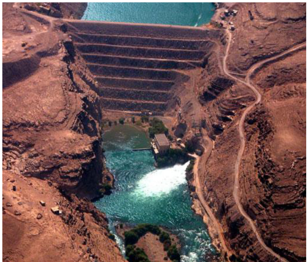
Figure 2: The Kajakai Dam, located in Southern Afghanistan on the Helmand River. Photo courtesy of the U.S. Army.
