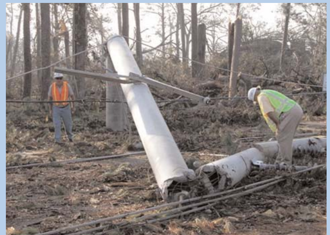
Utility crews examine a snapped pole during last year's hurricane season.
