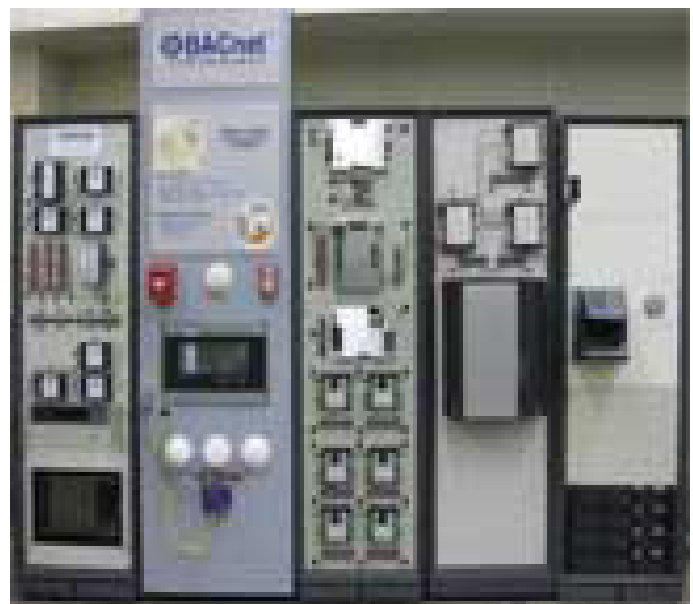
Embedded Intelligence in Buildings
