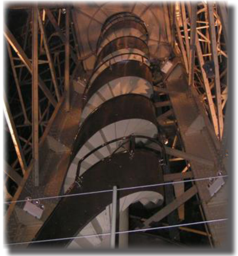
The double helix staircase inside the Statue of Liberty.
