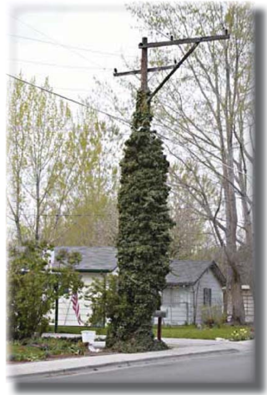
Vines growing on power poles are dangerous and illegal.
