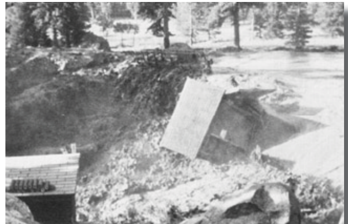
Lawn Lake Dam failure, Colorado. 1982
