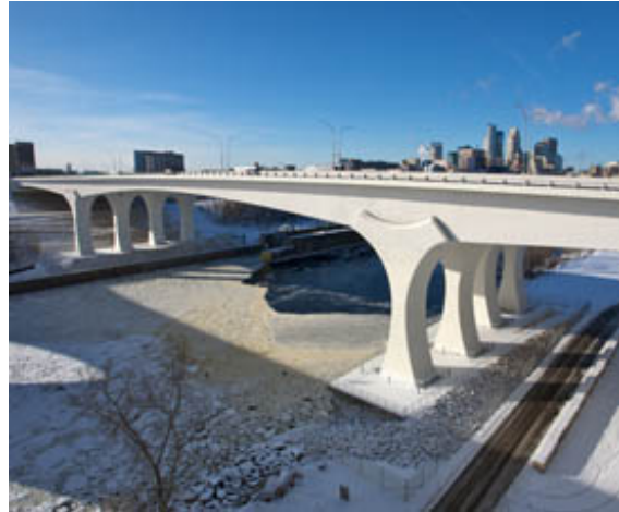
The St. Anthony Falls Bridge replaced the fallen I-35W Bridge in September 2008. Photo courtesy of the design-build firm Flatiron.
