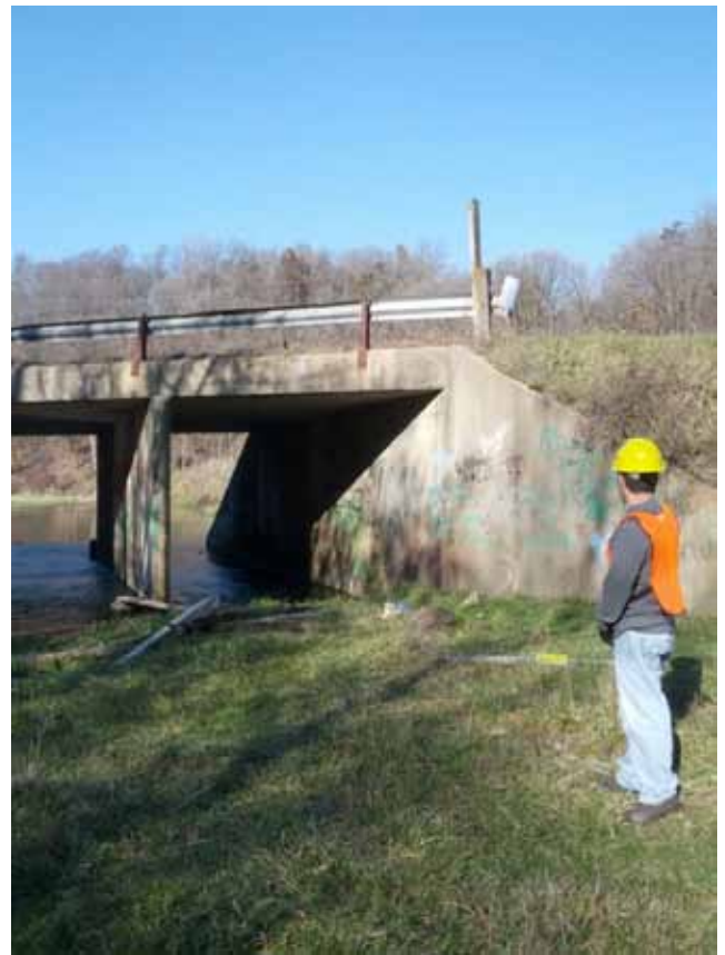
Figure 1. A student inspecting the condition of a rural bridge.
